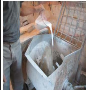
Photo 06: Liquid (mixed previously) being added to mortar mix.
