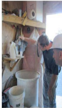
Photo 04: Liquid composed of 50% restoration latex RL1 by Edison Coating Inc. and 50% potable water is to be measured carefully separately before.
