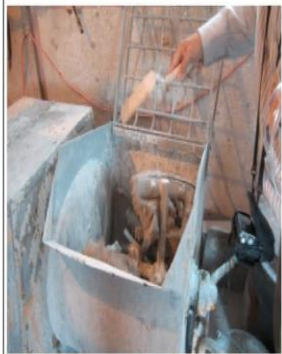
Photo 12: Contractor to make sure mortar doesn't stick to the mixer's paddles when mixing.
